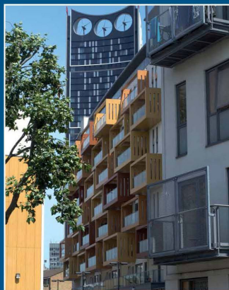
New homes in Strata and Crampton Street
